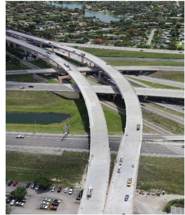
SR 874 Northbound/Southbound Connector Bridges to SR 874
